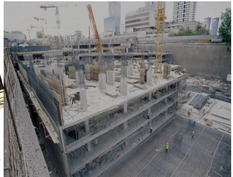
RESIDENCE CONSTRUCTION 29 FLOORS ERBIL - IRAQ
