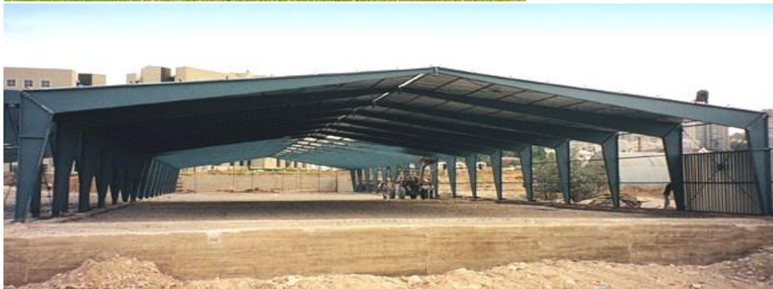
WARE HOUSE BUILDING
